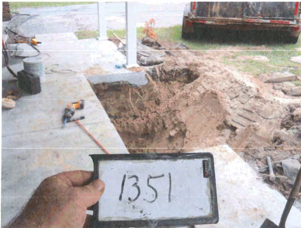
Picture 2: UST 1351 Cardinal excavation.
